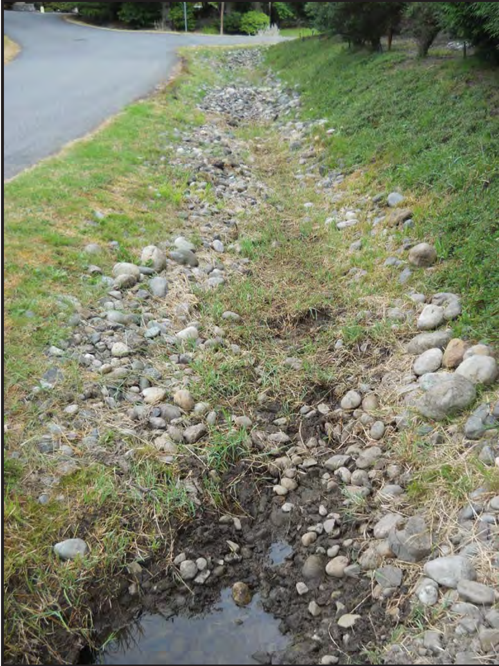
Channel downstream of culvert outlet.
