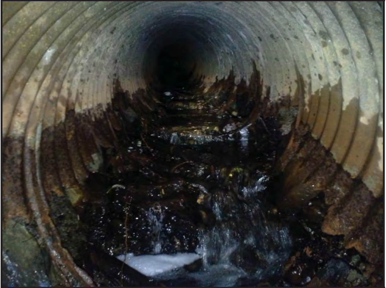
Culvert barrel at outlet.
