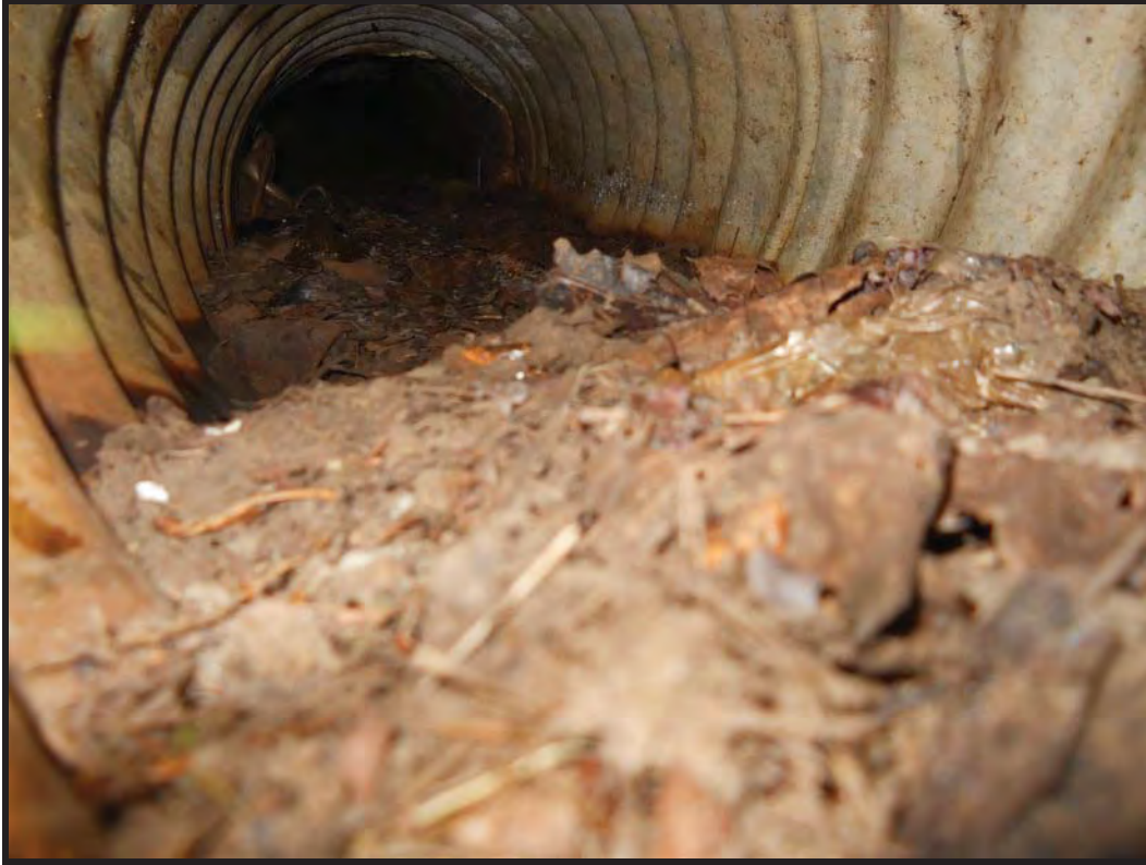
Culvert barrel at inlet.
