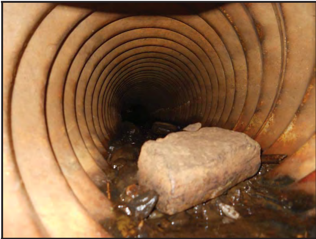
Culvert barrel at inlet.
