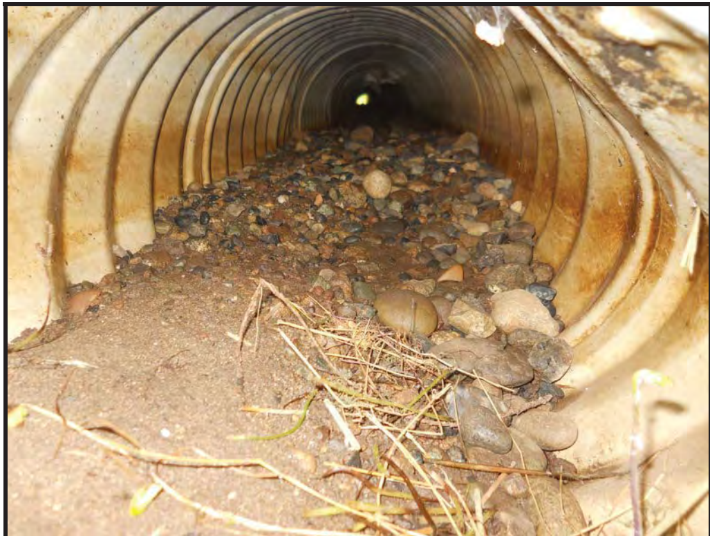
Looking down culvert barrel from inlet.
