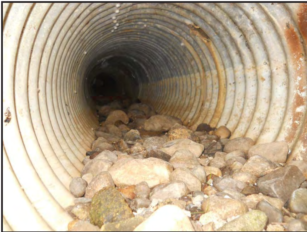
Culvert 213 barrel at outlet.
