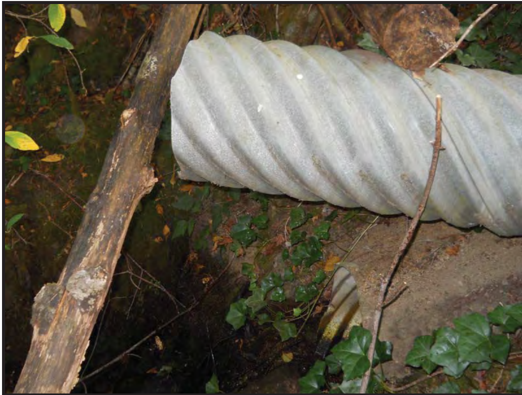
Culvert outlet (below) - additional pipe outlet directly above.
