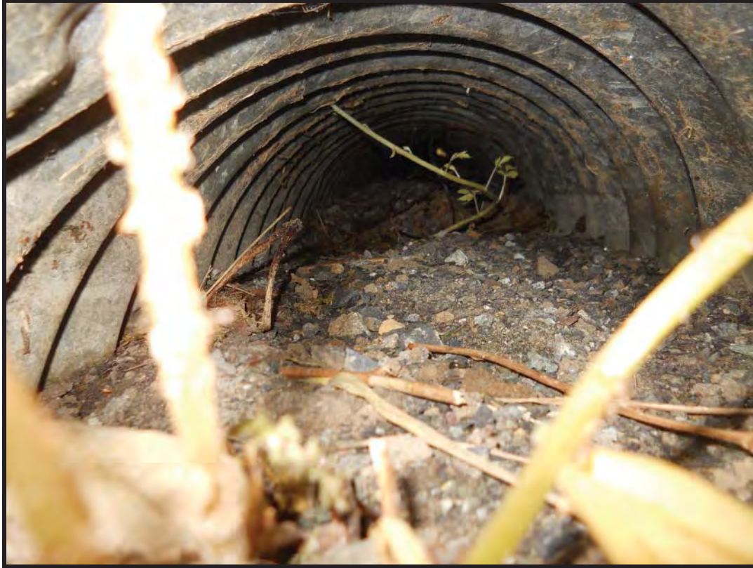
Culvert 212 barrel at outlet.
