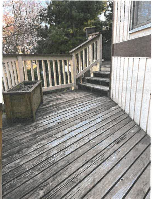
Existing Wood Deck & Railing
