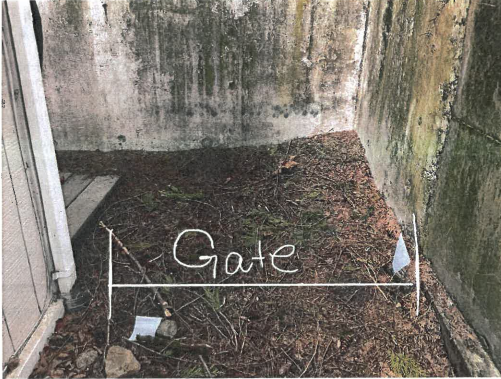
This is the right side of house (from street) to completely enclose the backyard dog run.
