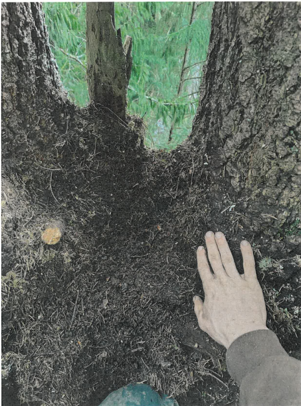
Figure 4. Interior of the bifurcation showing accumulated decayed wood and organic debris. The dead top is assumed to have decayed downward into the union. Hand for scale.
