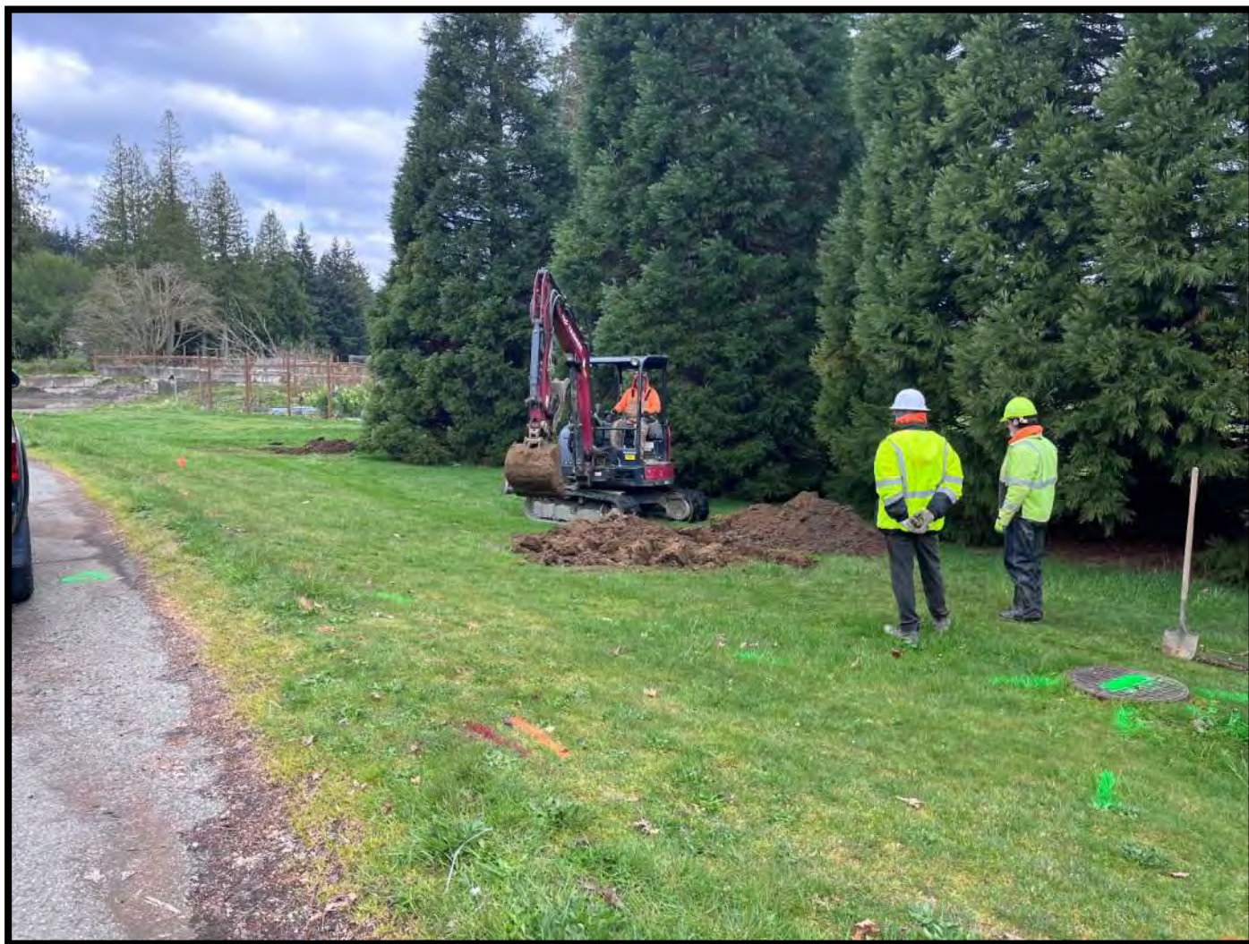
Photo 8: Test location TP-8 in progress N of the asphalt pavement and barn facility. Facing W on April 16, 2026.
