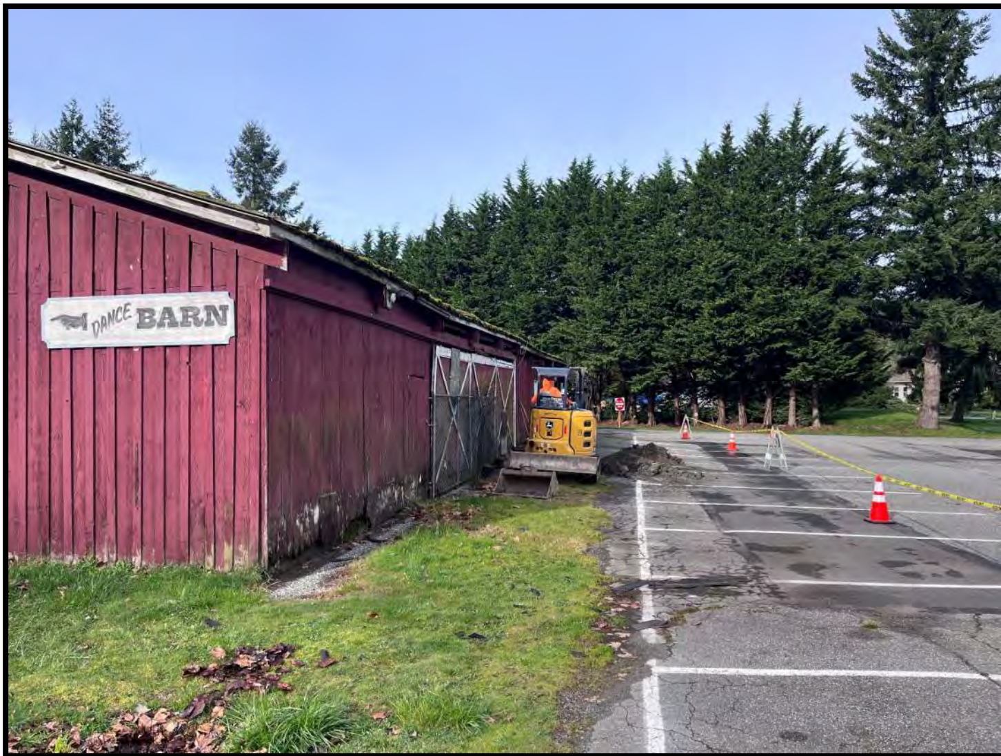
Photo 2: The N side of the barn with TP-1 in progress on March 27, 2026.
