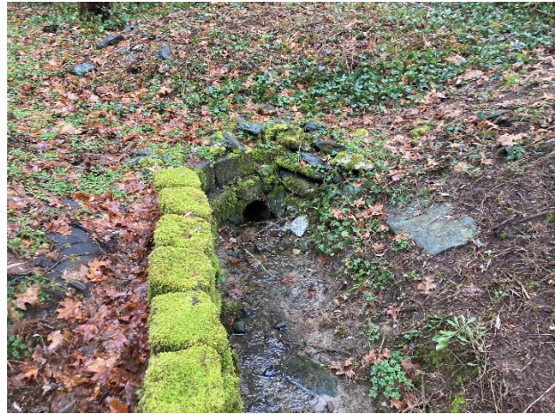
Above – 8” culvert that is unmapped and drains to Beaver Creek.
