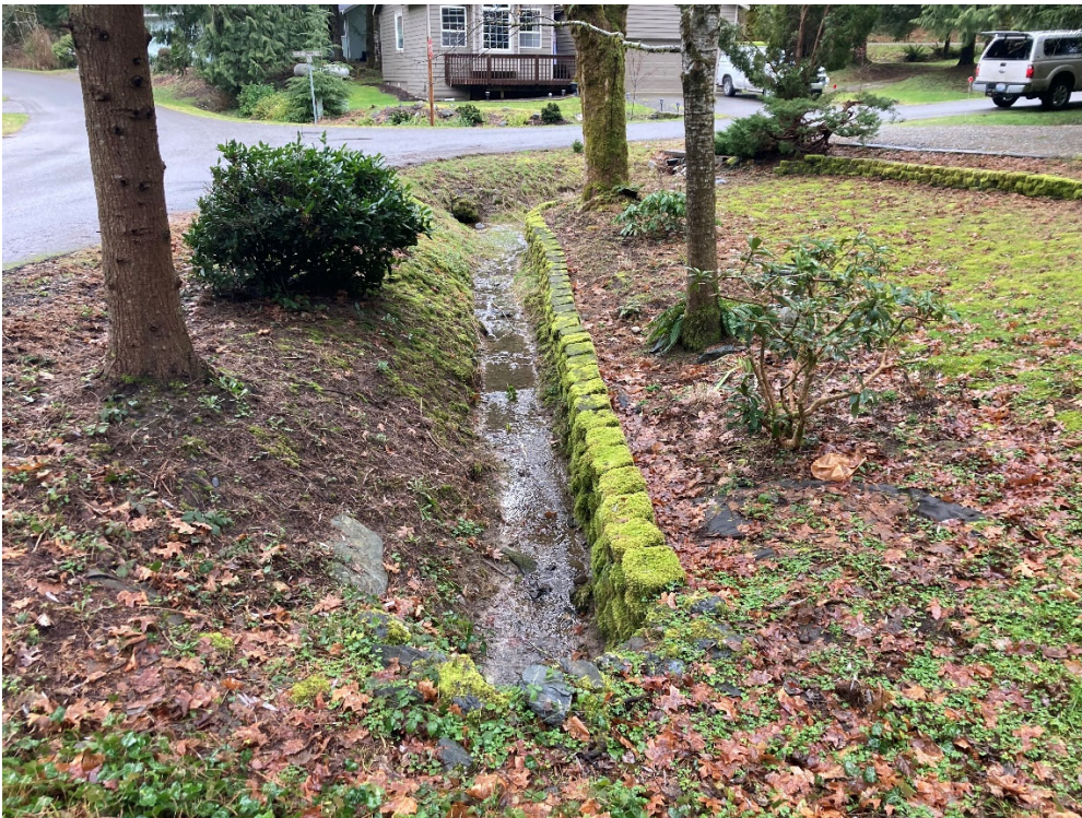
Below – Ditch leading to 8” culvert, and 12” culvert 208 crosses under road.
