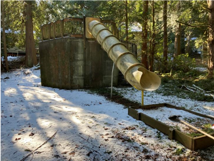
Treehouse Park structure (1)
