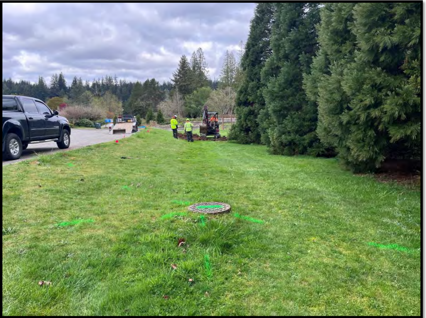
Photo 7: Test location TP-7 in progress N of the asphalt pavement and barn facility. Facing W on April 16, 2026.
