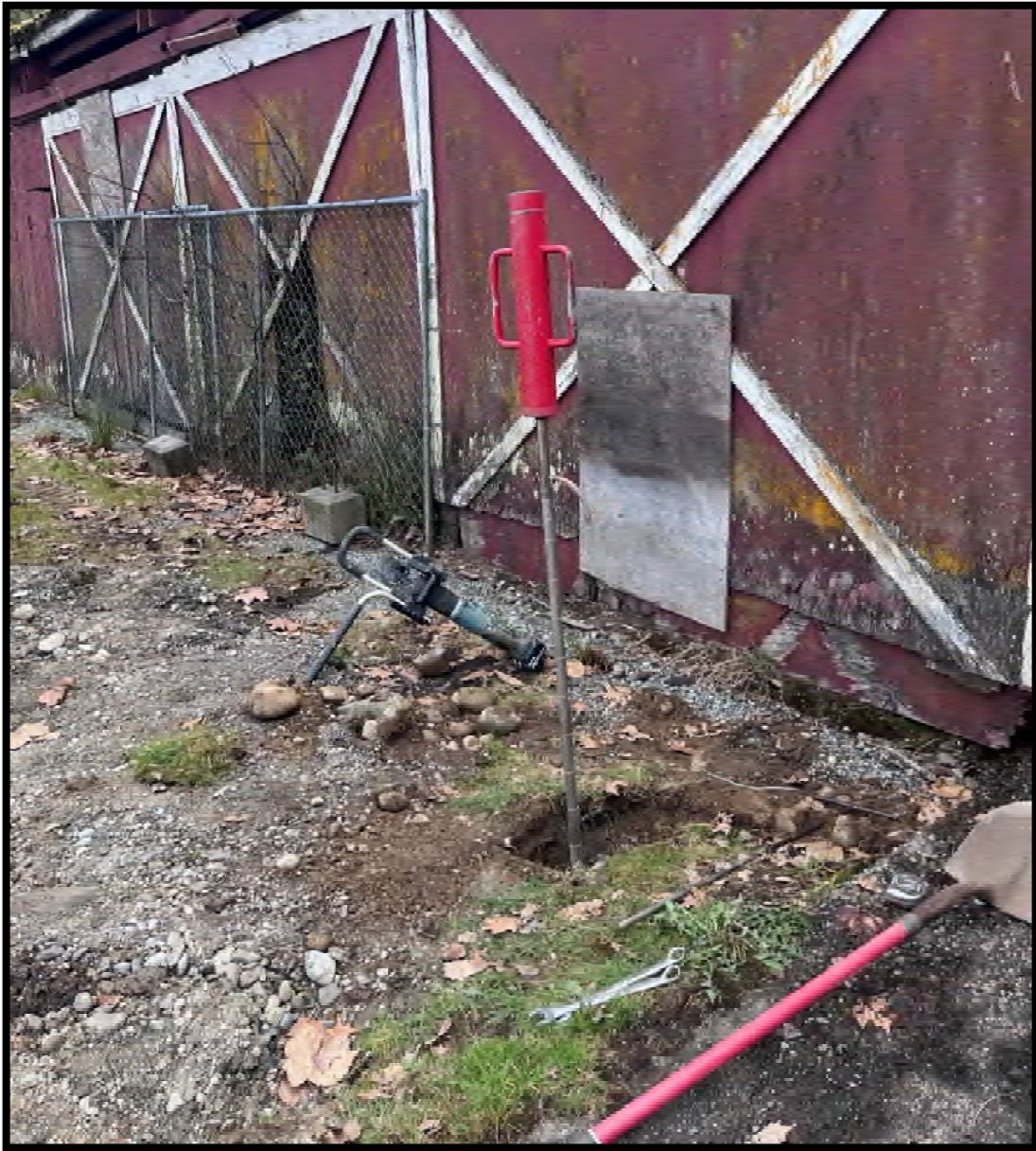
Photo 5: Test location DCP-1 in progress adjacent to TP-1. Facing SE on April 10, 2026.
