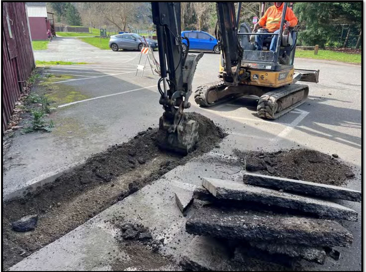
Photo 4: Test location TP-4 in progress on the W side of the barn. Facing S on March 27, 2026.
