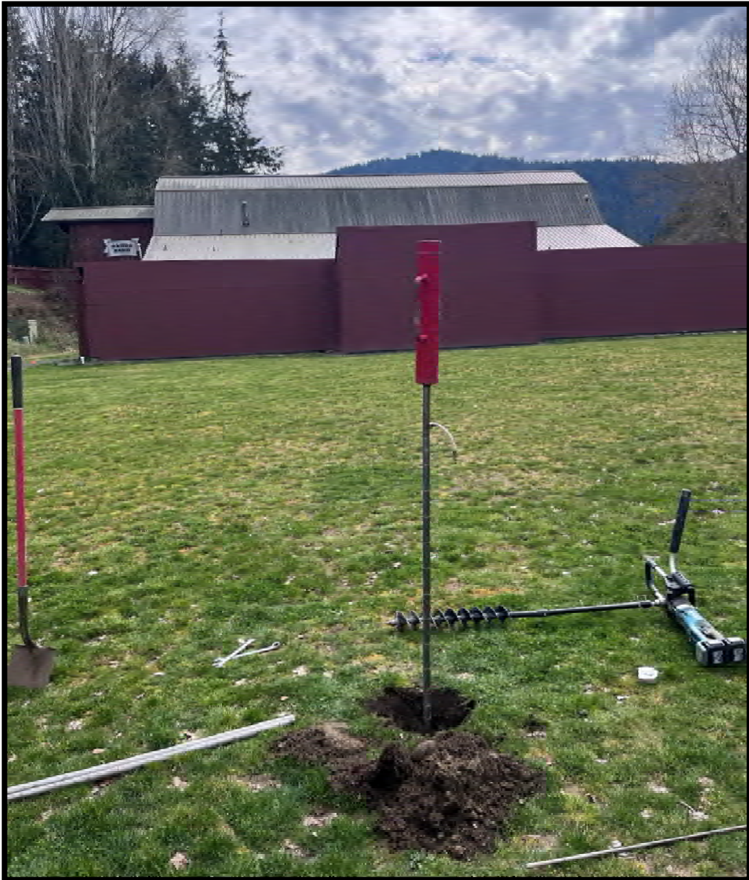
Photo 6: Test location DCP-2 in progress on the S side of the barn. Facing S on April 10, 2026.
