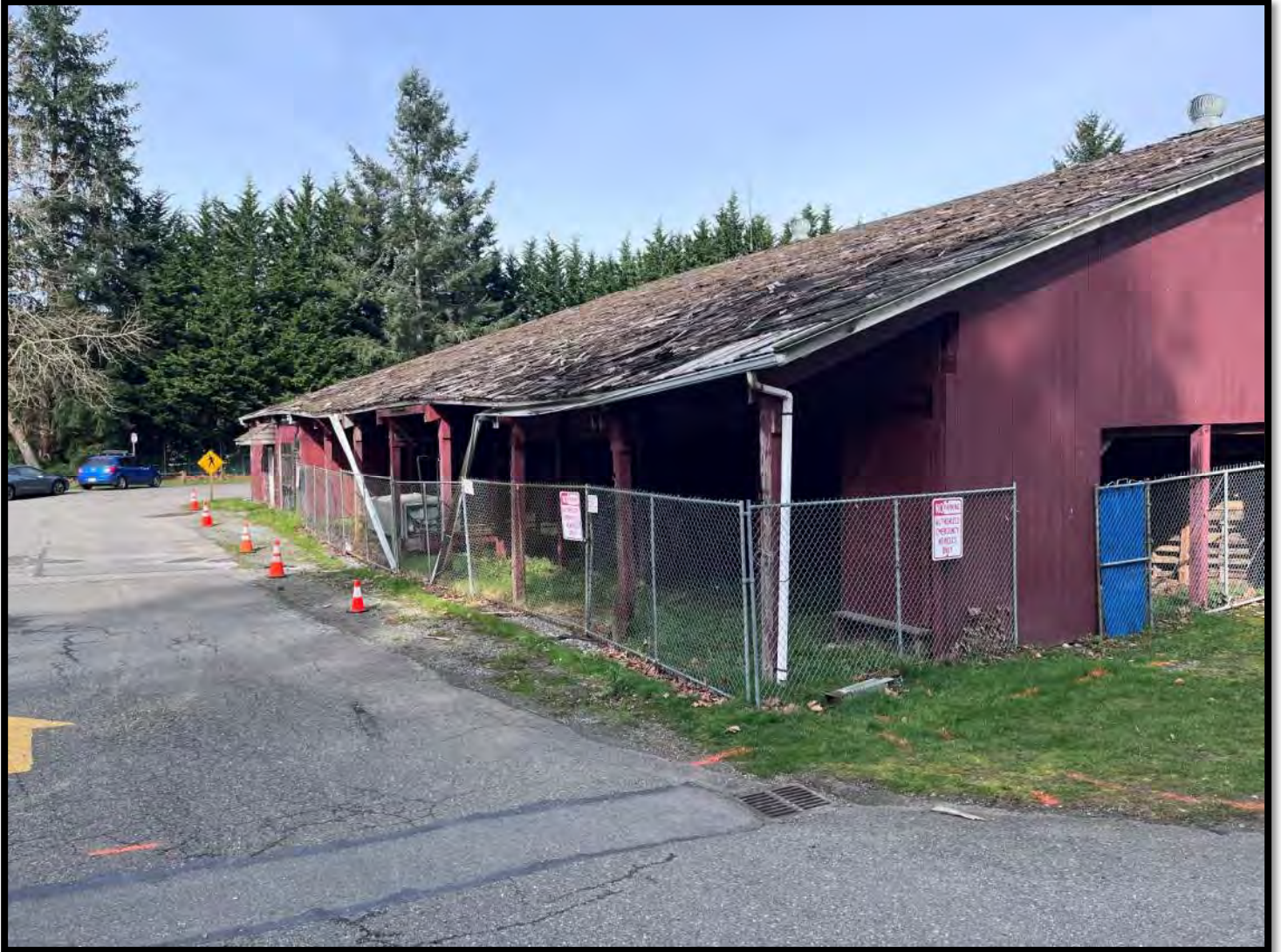
Photo 3: The S side of the barn, facing W on March 27, 2026.
