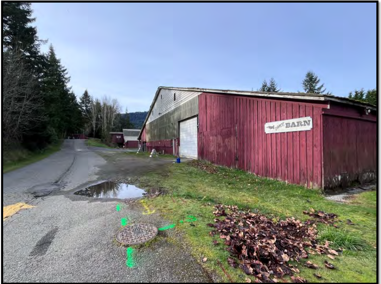
Photo 1: Existing conditions at the barn facing S on March 27, 2026.
