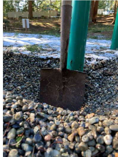
Cascade Park surfacing (1)
