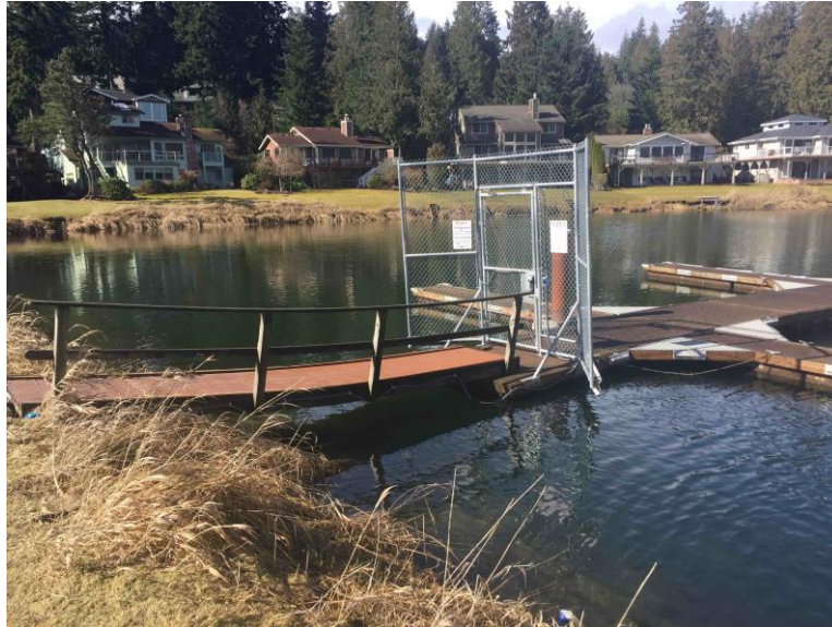
Photo 11, West Dock gangway
