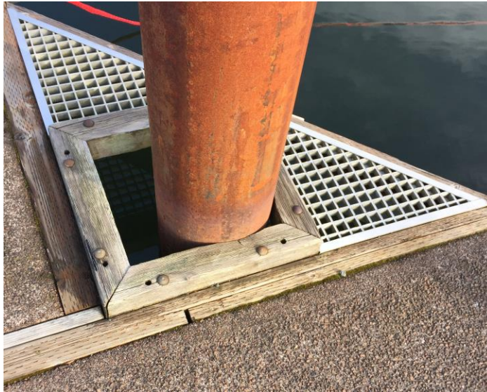
Photo 9, Triangle frame with pile guide.
