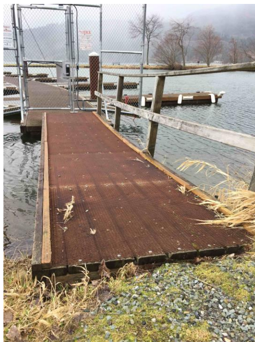
Photo 10, East Dock gangway
