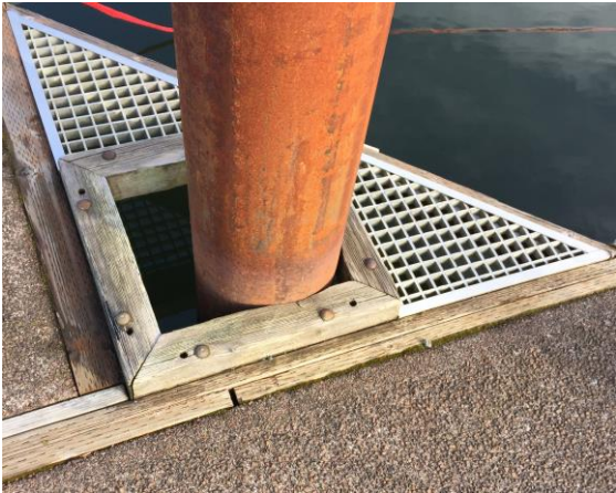
Photo 6, Triangle frame with pile guide.
