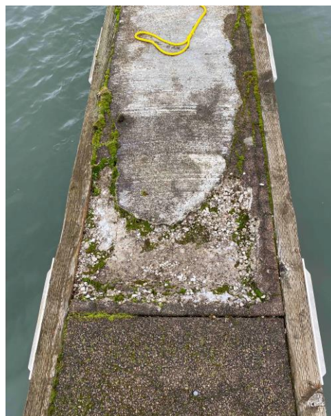
Photos 1 & 2 Deck damage at Slip 72 East Dock.
