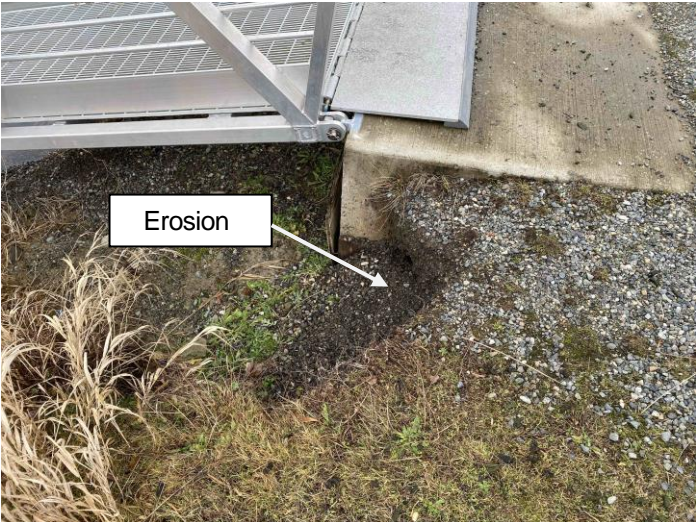
Photo 8, West side of the West Dock abutment
