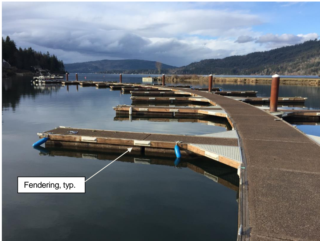
Photo 1, Typical fendering
