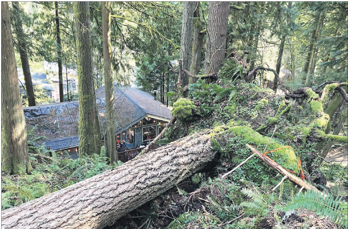
On April 10, the SVCA Board approved CRRRF money to pay for removal of a hazardous tree at 12 Sudden Valley Drive. The $40,000 expenditure will also cover mitigation of the risk of loose boulders, as well as ensure site safety. (SVCA photo)
